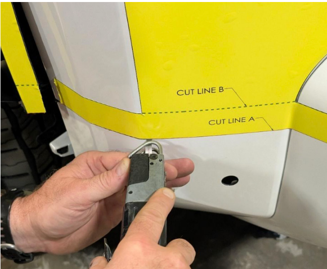
Figure 41 – Cutting Fascia with Template
